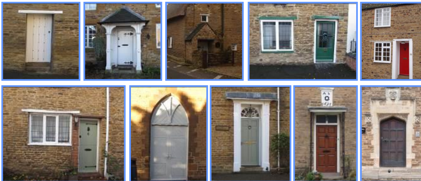
Figure 47 Examples of traditional doors in the conservation area. Traditional doors are made of timber, and are variously plank or panel, occasionally with small glass panes or fanlights.
