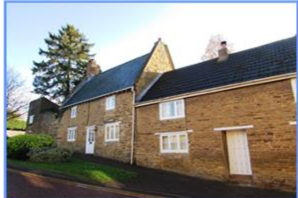
Figure 42 The steeply pitched projecting gable of this building denotes previous thatching. Its shape enhances the character of the street.
