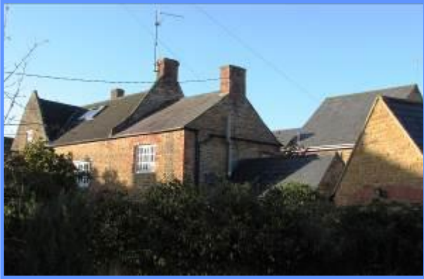
Figure 43 Ridgelines may be seen from many angles, leading to lively character and the need for sensitive development.
