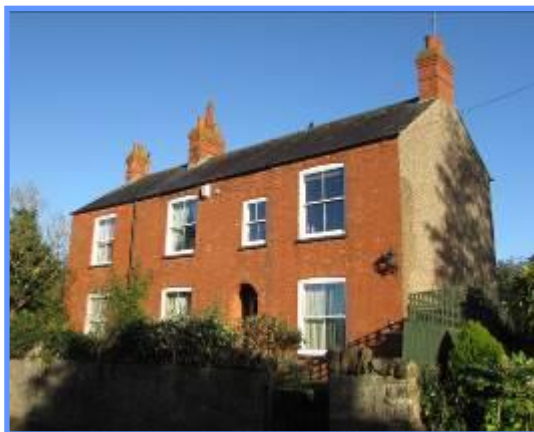
Figure 35 Brick Victorian villa on Northampton Lane North.
