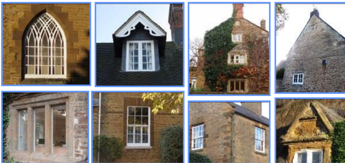
Figure 46 Examples of historic windows within the conservation area. They are mainly timber framed, but the style varies depending on the use and type of building.
