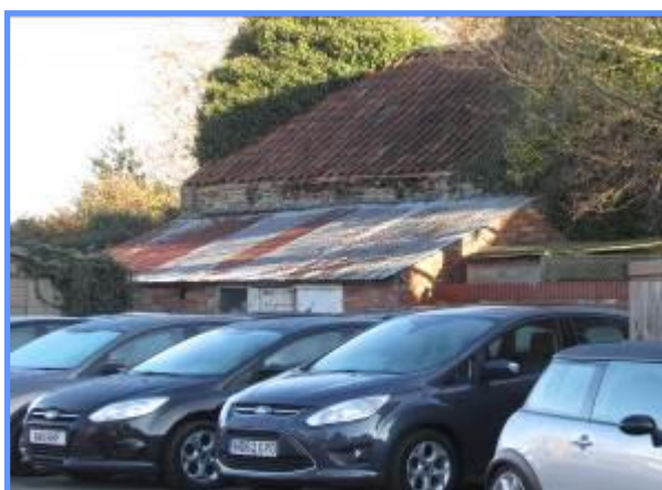
Figure 40 Pantiles are used throughout the village on outbuildings, as here, along with corrugated tin, a local style.
